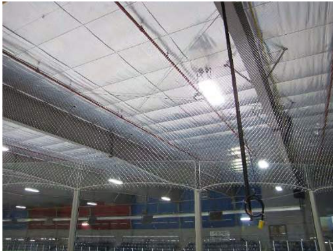
Arena low-e ceiling in excellent shape
