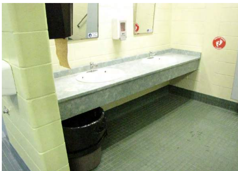
Washroom counter requires under cut to be accessible
