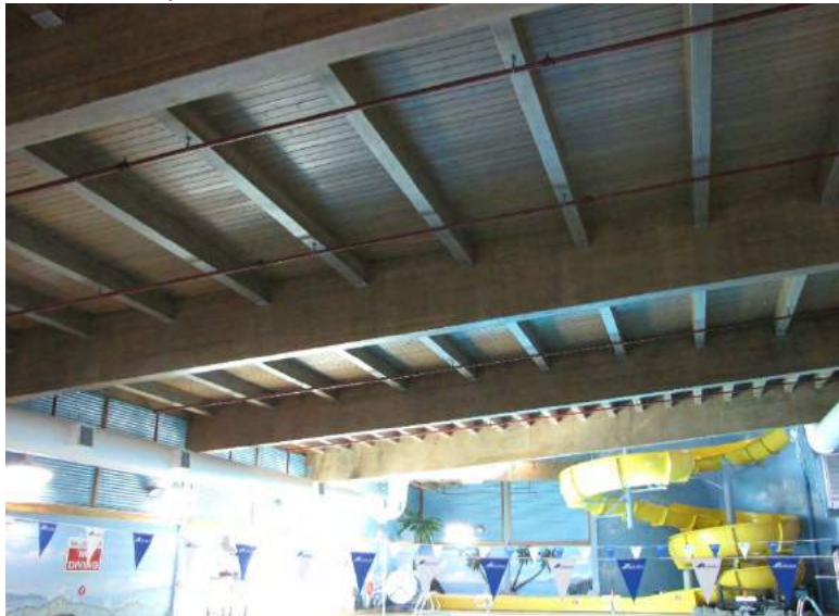
Wood beam structure and wood decking
