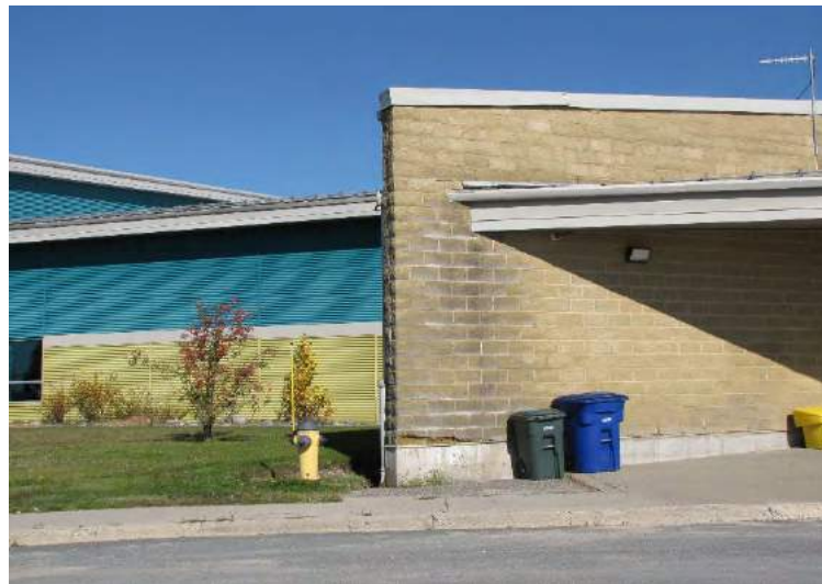
Edge of canopy and supporting structure, water damage to the Block, flashing / repair required.
